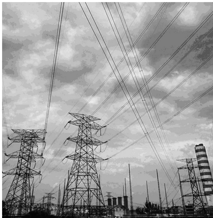
FIGURE 47.5 Transmission lines out of Connaught Bridge Power Station, Malaysia.
