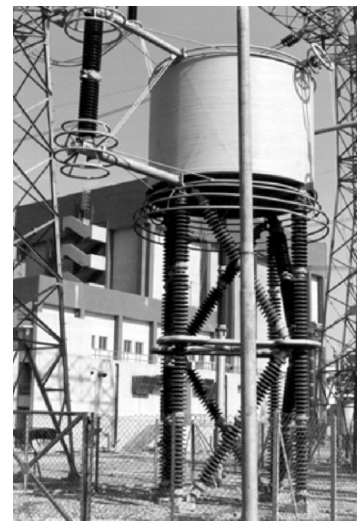
FIGURE 31.8 Installation of an air-cooled smoothing reactor.
